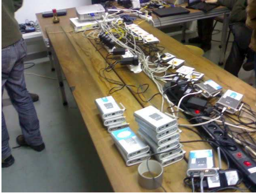
Photo above : Table with the hardware nodes freshly flashed (Kamikaze r18470 with minimal packages) and connected to the switch and the configuration server.
